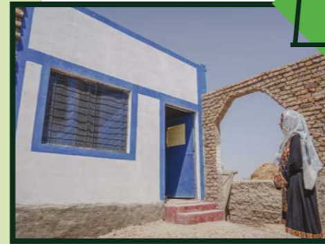
After the Pakistan floods of 2023, families received materials to construct a more durable shelter, including local limestone, known for its water-resistant properties.
